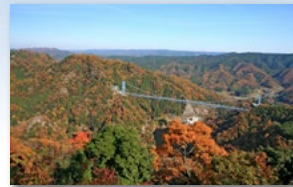
Ryujin Big Suspension Bridge
